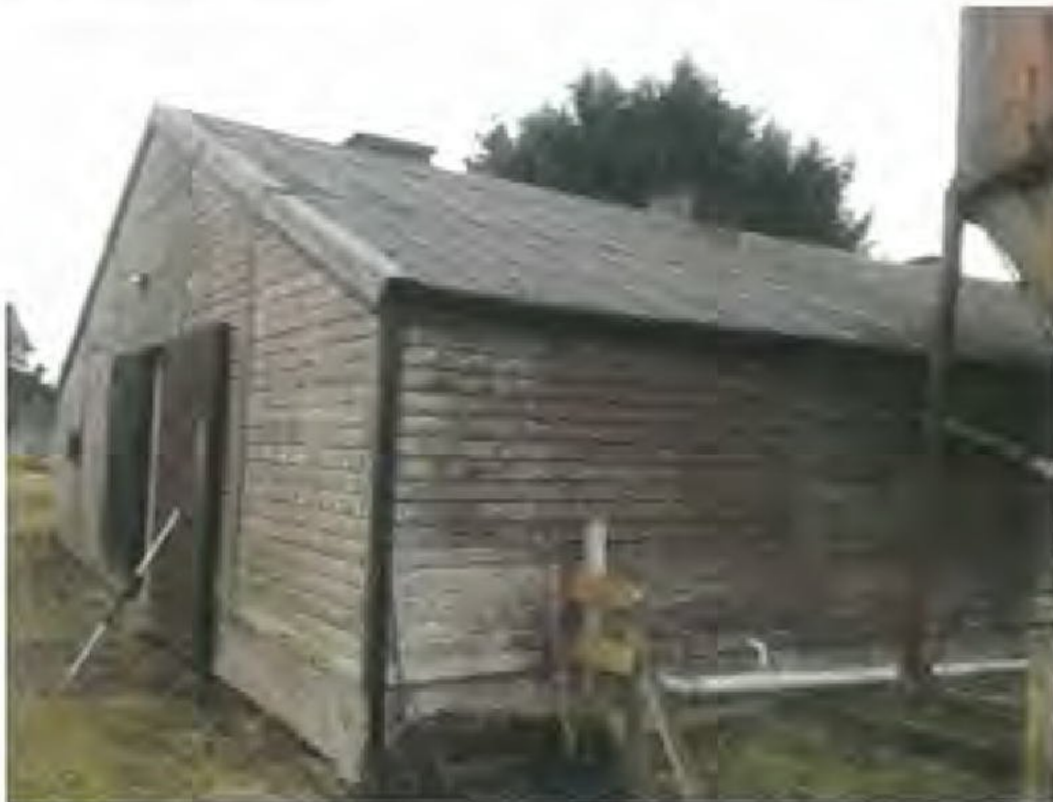
Figure 3. Photograph of front entrance of Poultry Unit shed (west elevation)
