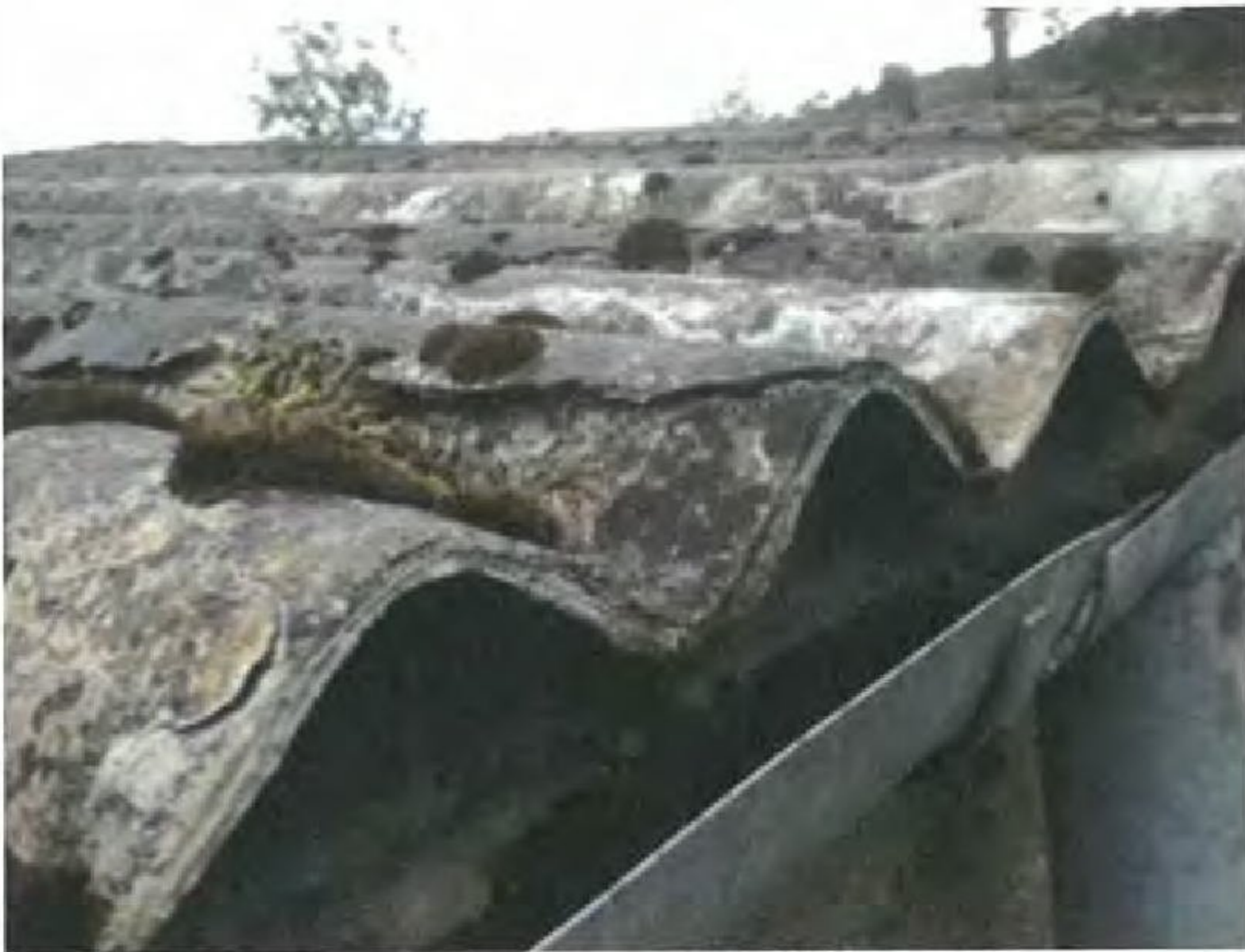
Figure 5. Asbestos cement roof sheeting to sheds [B] to west of site
