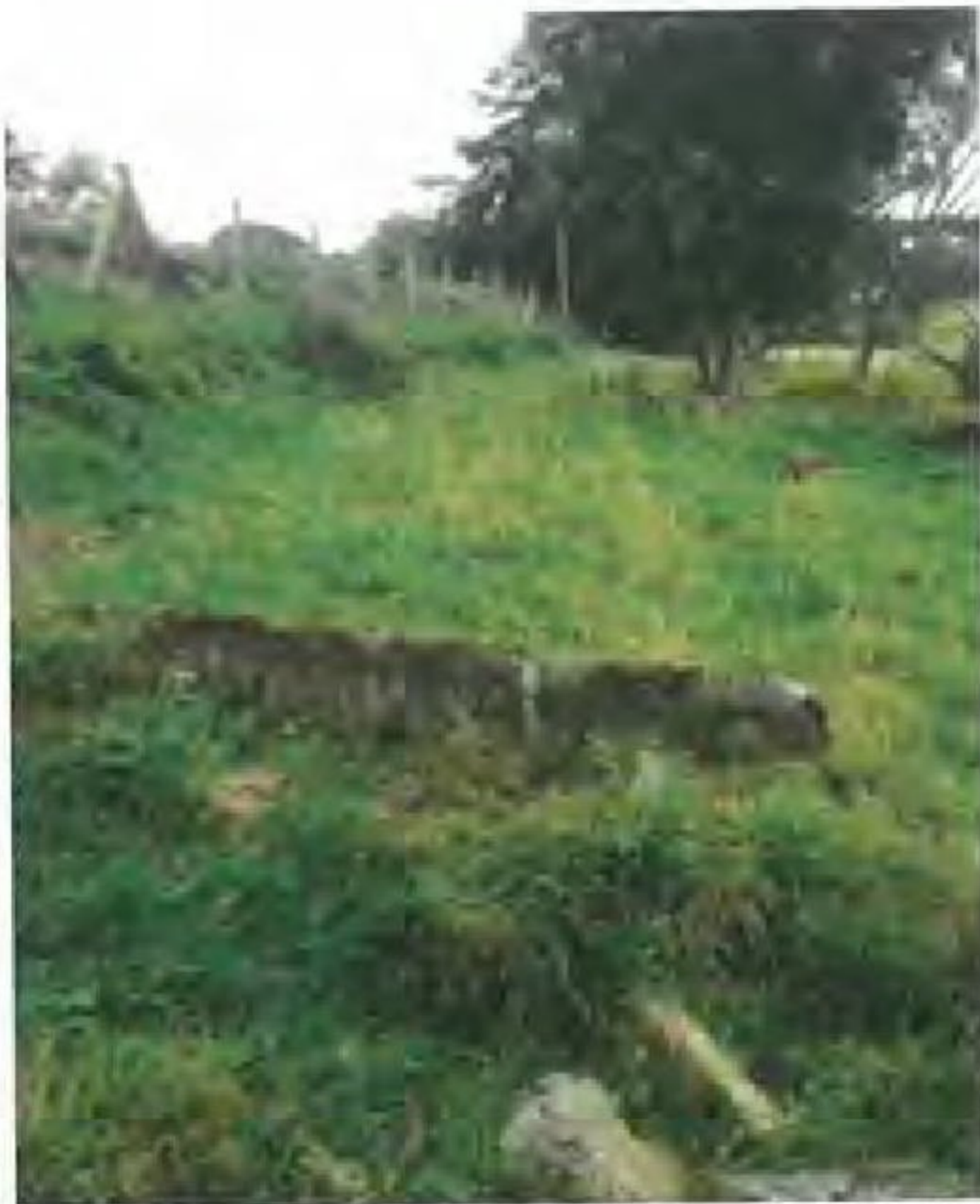
Figure 7. Footing to unknown structure to east of B, with asbestos cement sheeting within wall.
