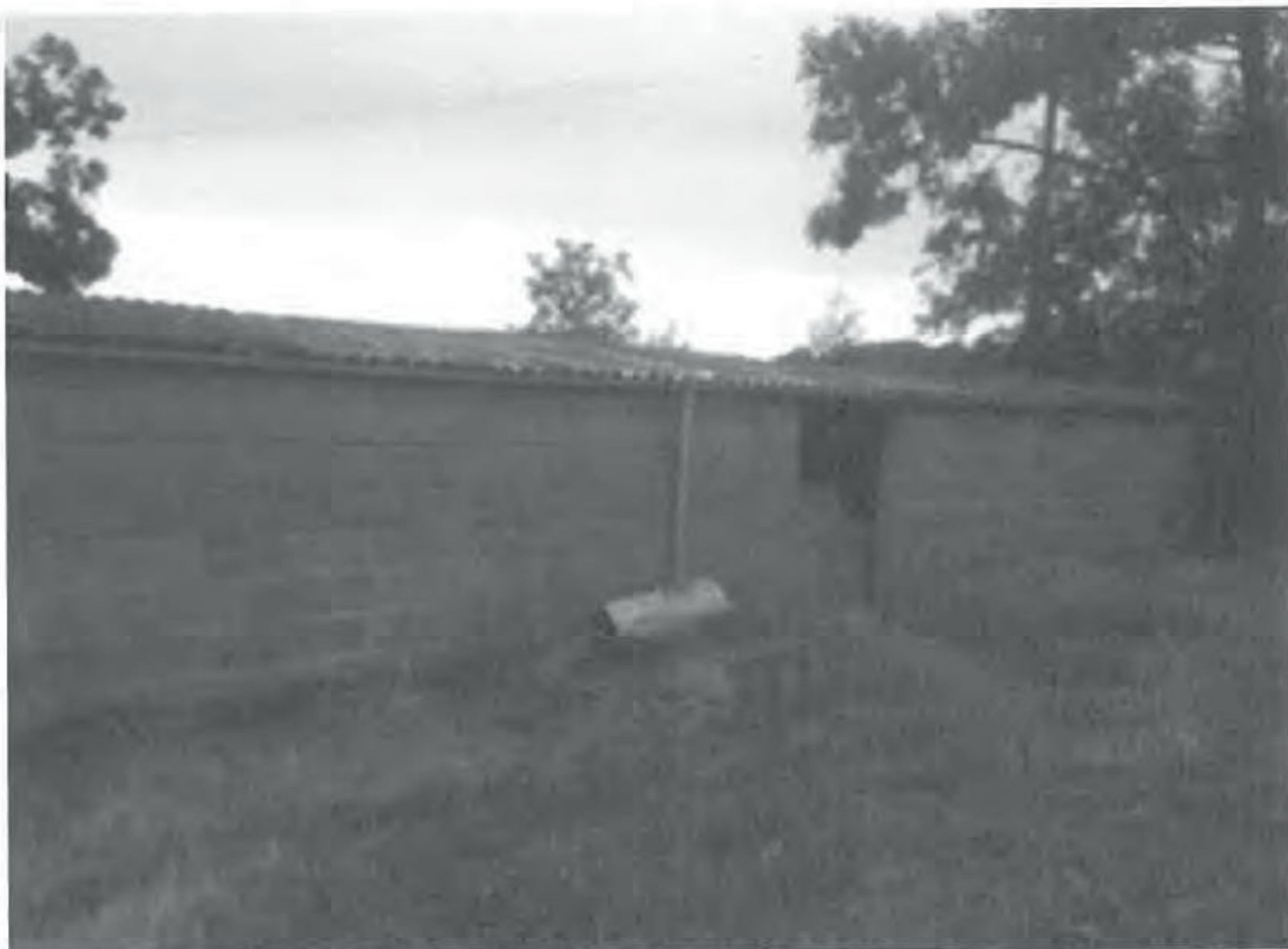
Figure 4. East Elevation of Sheds [B] to west of site
